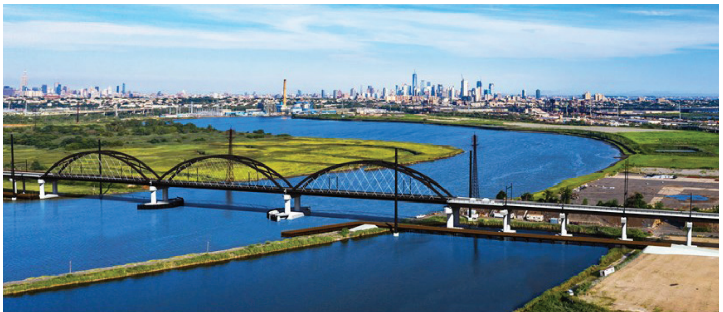
The Portal North Bridge replacement in New Jersey, USA
