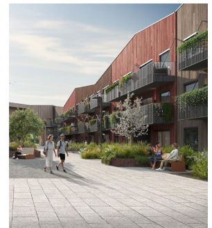
Powerhouse Lade, Trondheim, Norway
