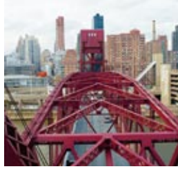
Roosevelt Island, located in New York City's East River, is reachable by car only via a lift span bridge constructed in 1955. The bridge – linking the borough of Queens with the island – has now been totally refurbished by Skanska, which received the assignment on the basis of its bridge expertise, not its price. The project was completed two months ahead of schedule.
