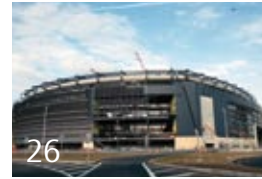
26 New technology for more efficient stadium construction
