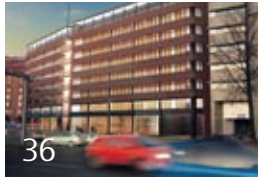
36 First LEED building in the Nordic countries
