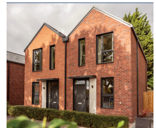
Residential development, BoKlok - On the brook, Bristol, UK
