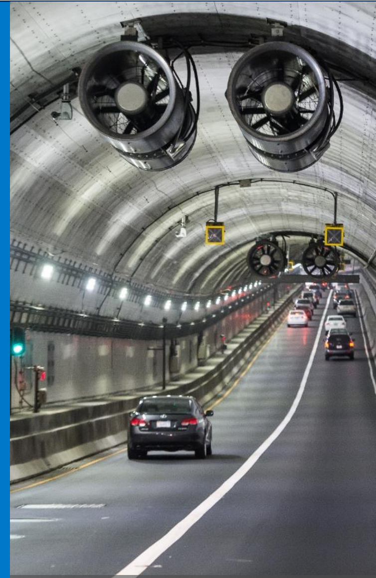
Elizabeth River Tunnels, Virginia, USA
