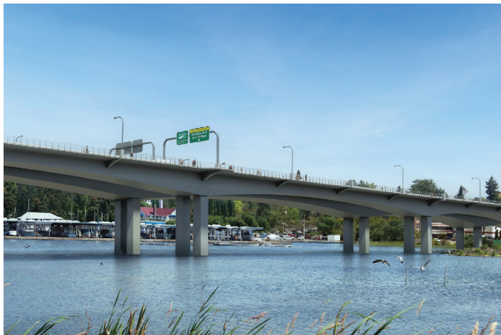
Portage Bay Bridge, Seattle, USA
