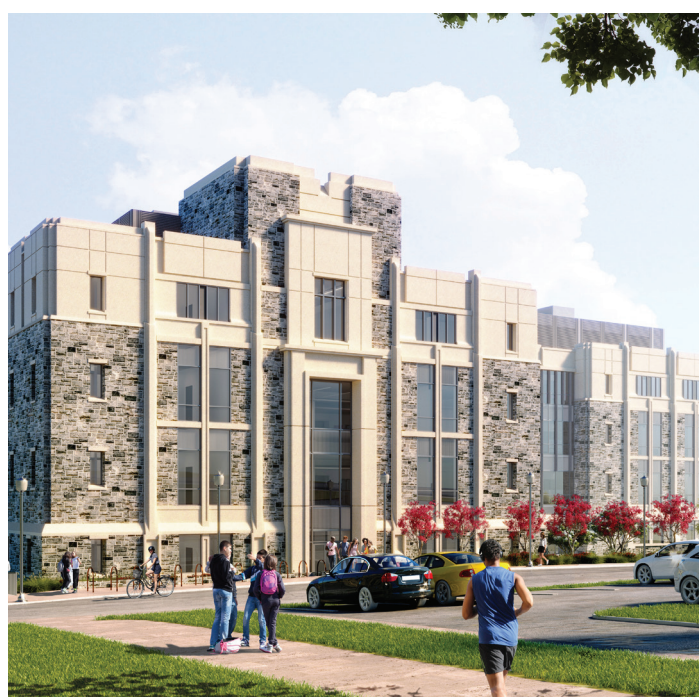
Undergraduate Science laboratory building, Blacksburg, Virginia, USA
