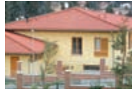
Single-family homes in Prague's outskirts 32
