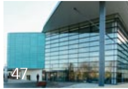
47 More than 1,100 beds at Derby City General Hospital
