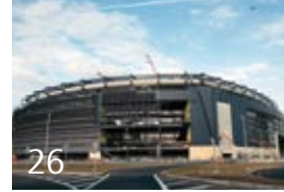
26 New technology for more efficient stadium construction
