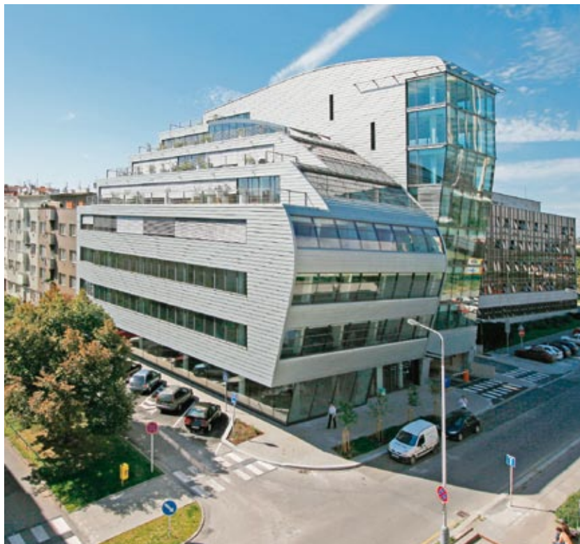
Vyšehrad Victoria is Skanska's latest commercial development project in Prague, Czech Republic. An architecturally distinctive project with 4,750 sq. m (51,000 sq. ft.) of office space. It offers green walk-on terraces as an extra amenity for tenants.
