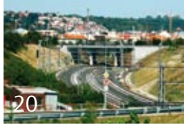
20 New railroad hub in Prague, Czech Republic
