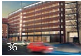
36 First LEED building in the Nordic countries
