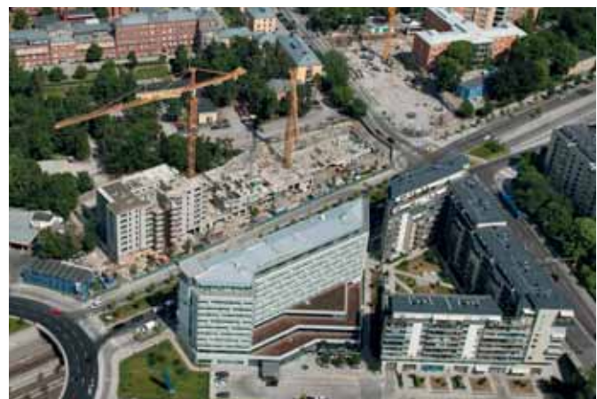
The Snöflingan and Iskristallen residential projects and the Courtyard by Marriott hotel, Stockholm, Sweden.
