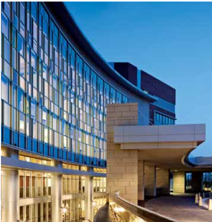
Hospital for Capital Health, Pennington, New Jersey, U.S.A.
