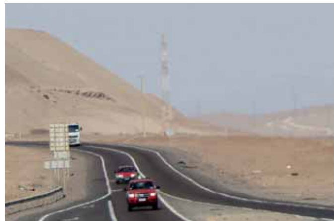
Construction of a new 120 km (75 mi.) long section of highway in Antofagasta, Chile.
