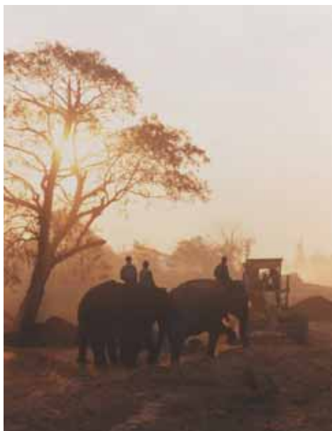
1994 Construction of a main highway in Laos.
