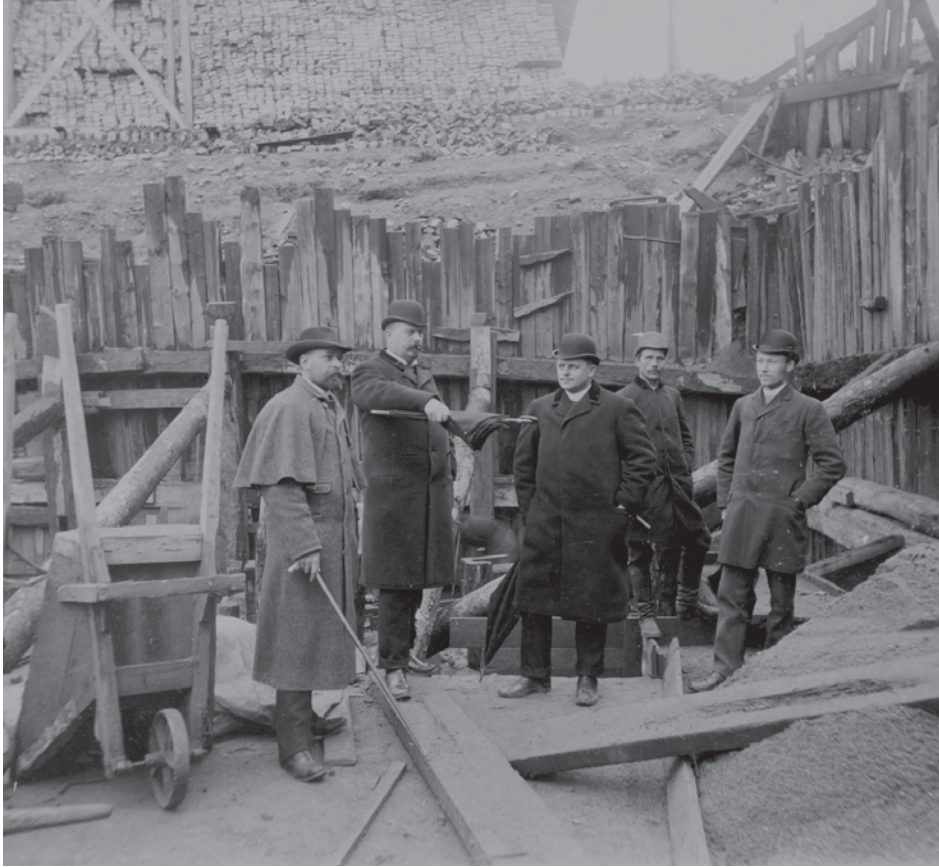
1899 Even today, the Royal Opera House in Stockholm stands on Skanska's solid concrete foundation.
