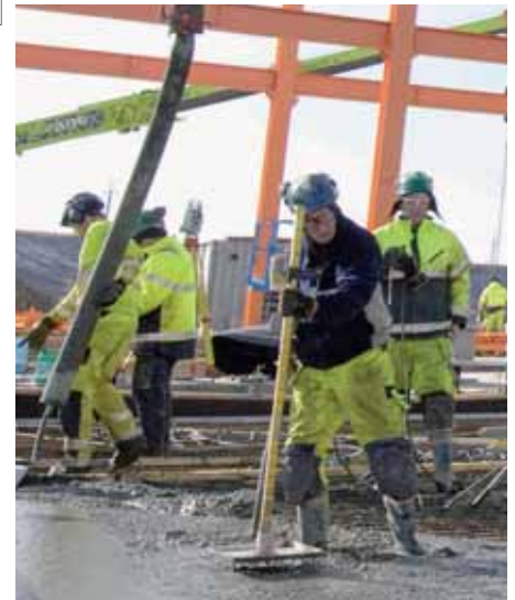
Up to 1,500 people are working on the construction of New Karolinska Solna in Stockholm, Sweden.
