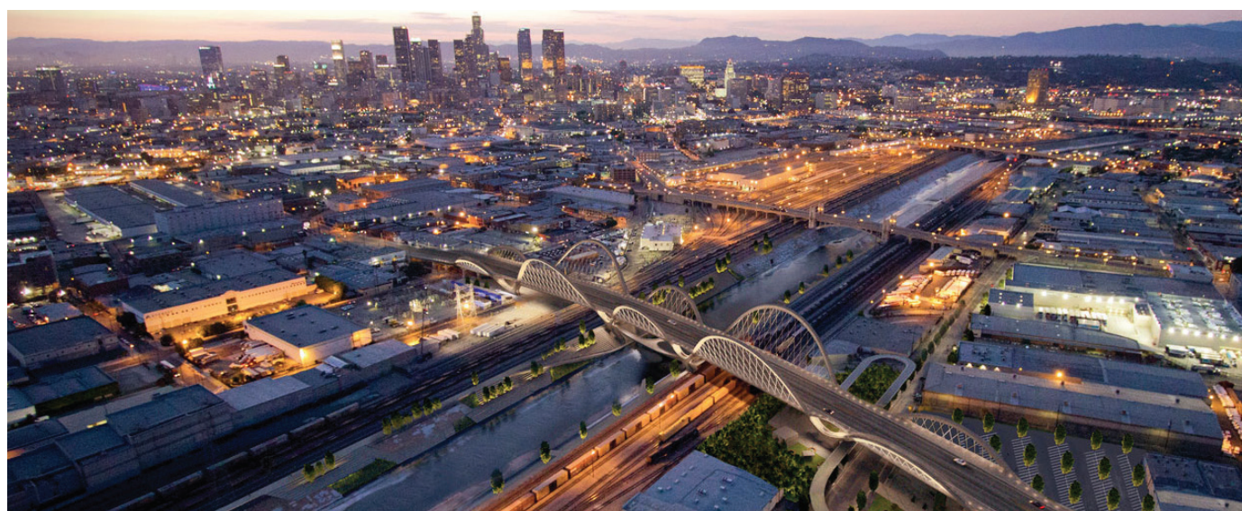
6th Street Viaduct, Los Angeles, USA.
