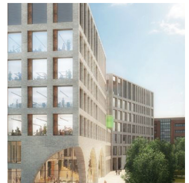
The Urban Environment House, Helsinki, Finland.
