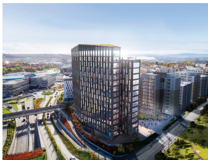
Investment in office project Parallell, Oslo, Norway.
