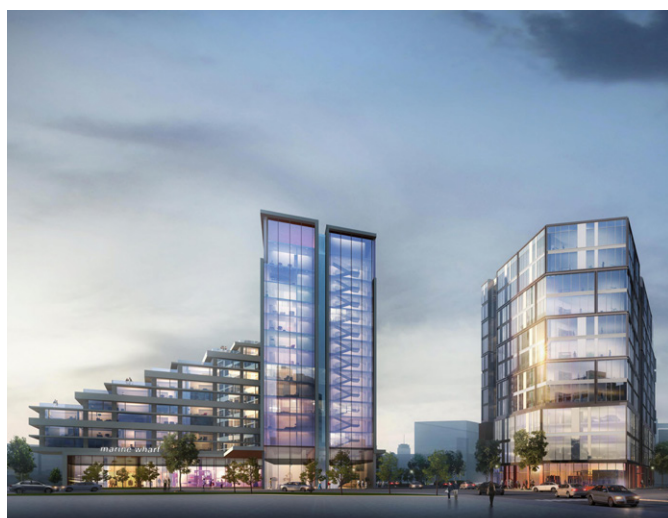
Investment in Drydock, Boston Seaport, Boston, USA.
