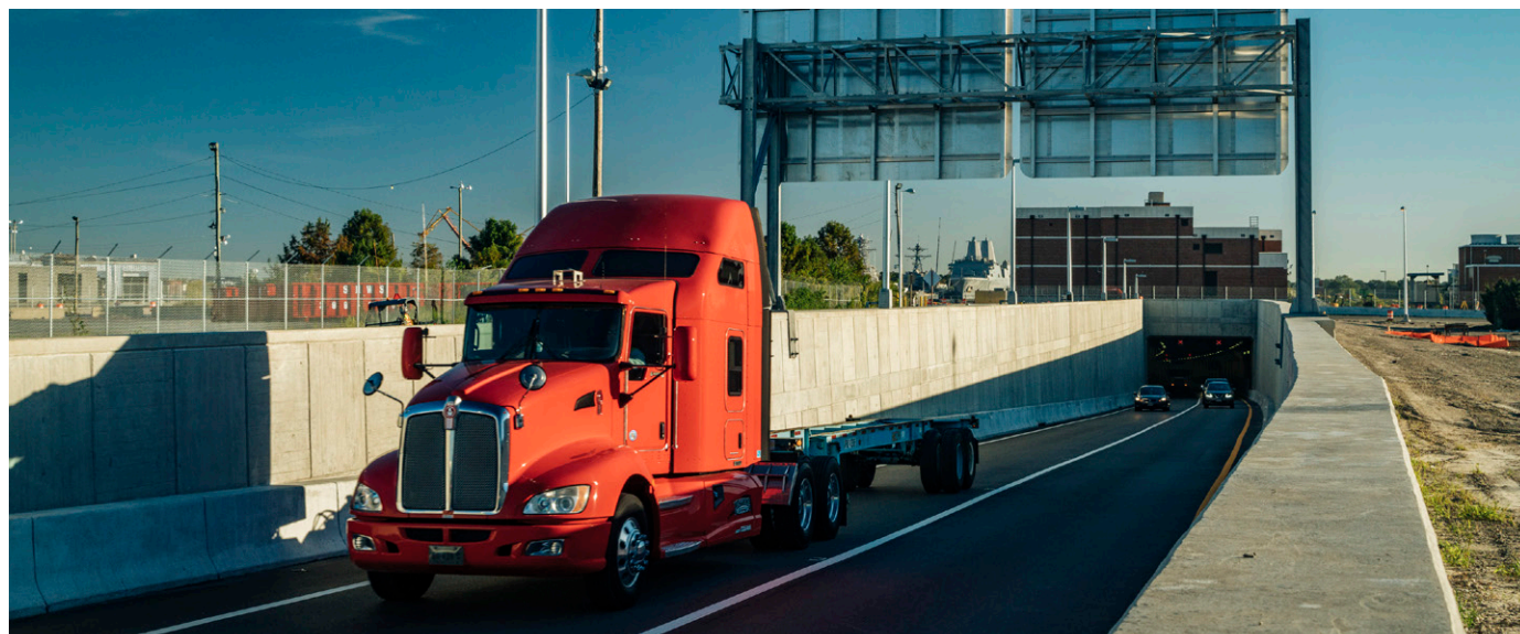
Elizabeth River Tunnels, Virginia, USA.
