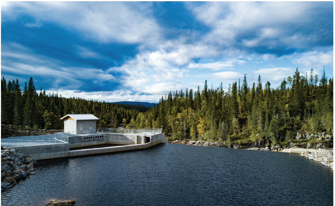
Storåselva, hydroelectric power plant, Hedmark, Norway.
