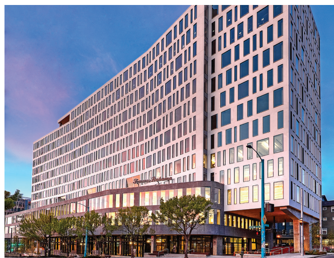
Divestment, Fairview 400, Seattle, USA.
