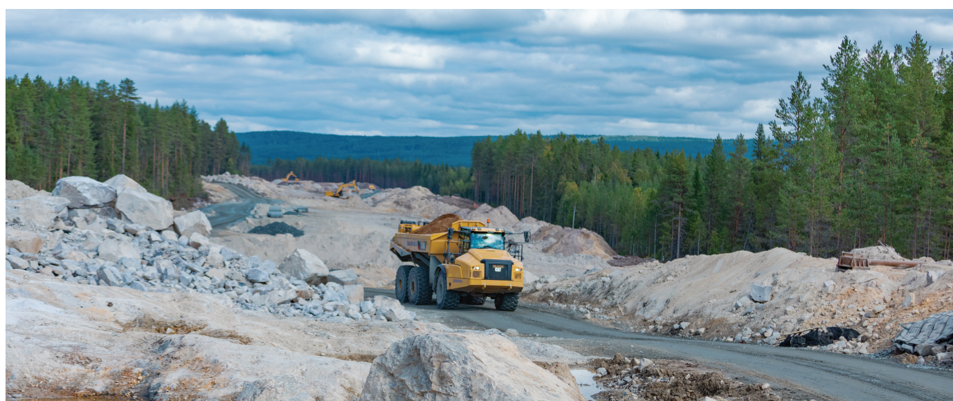
Rv3, road project, Løten to Elverum, Norway.
