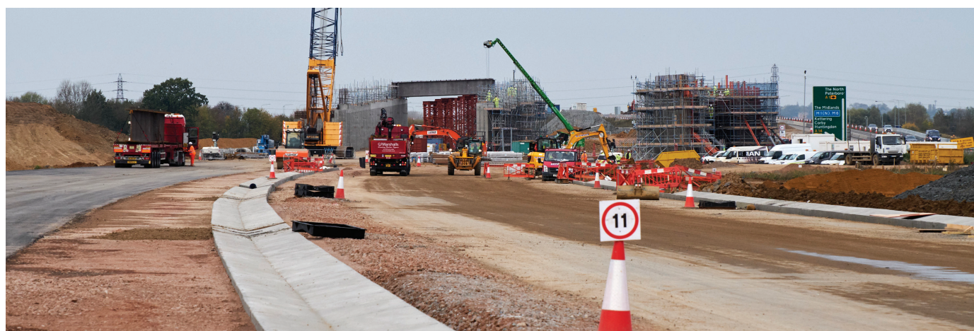
A14, highway project, Cambridge to Huntingdon, UK.
