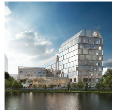
Office buildings, Jönköping, Sweden.
