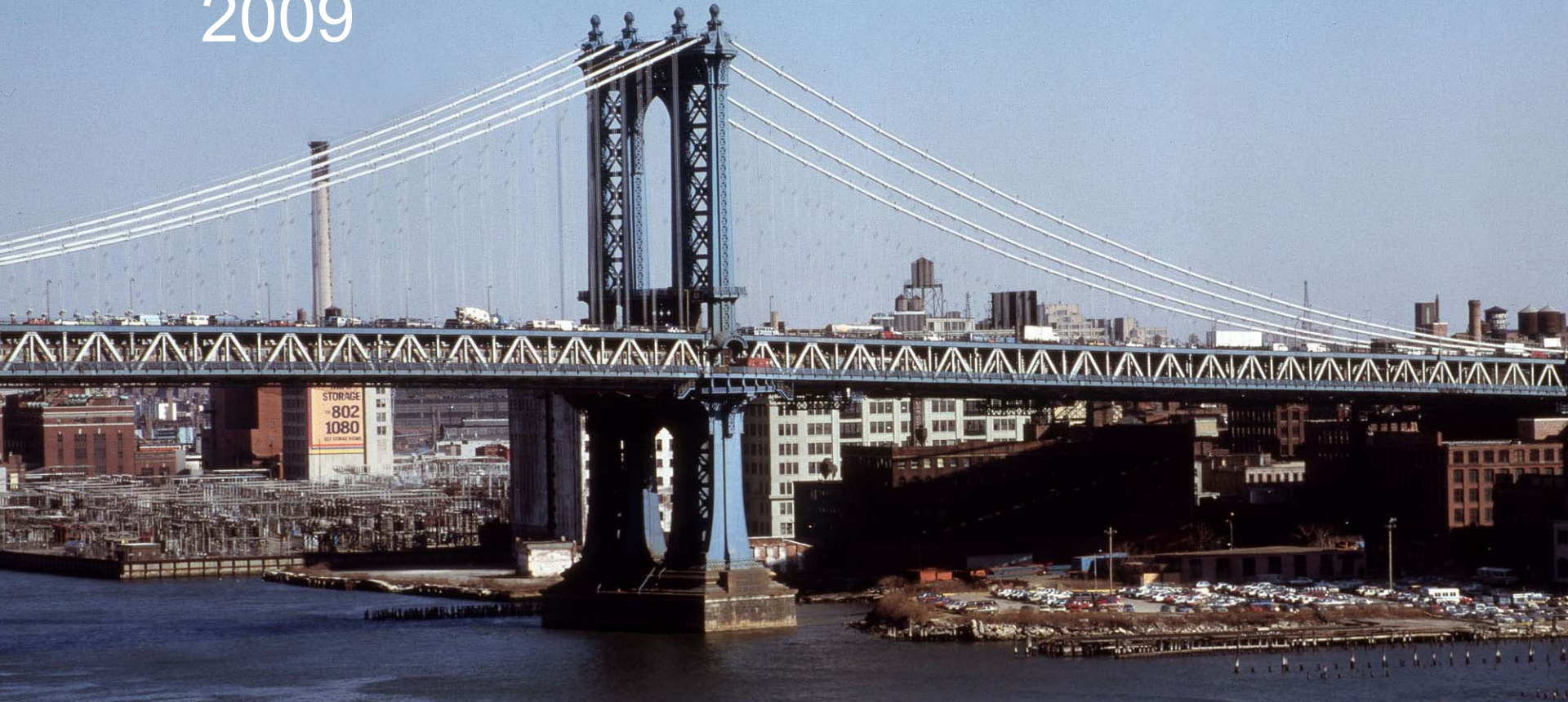
Manhattan Bridge, New York
