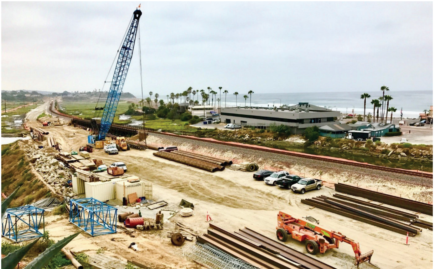
Phase 1 of Interstate 5 North Coast Corridor expansion project, San Diego, USA
