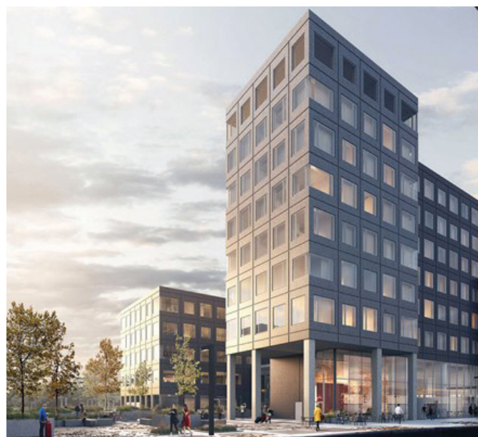
Investment, Ørestad City, Copenhagen, Denmark
