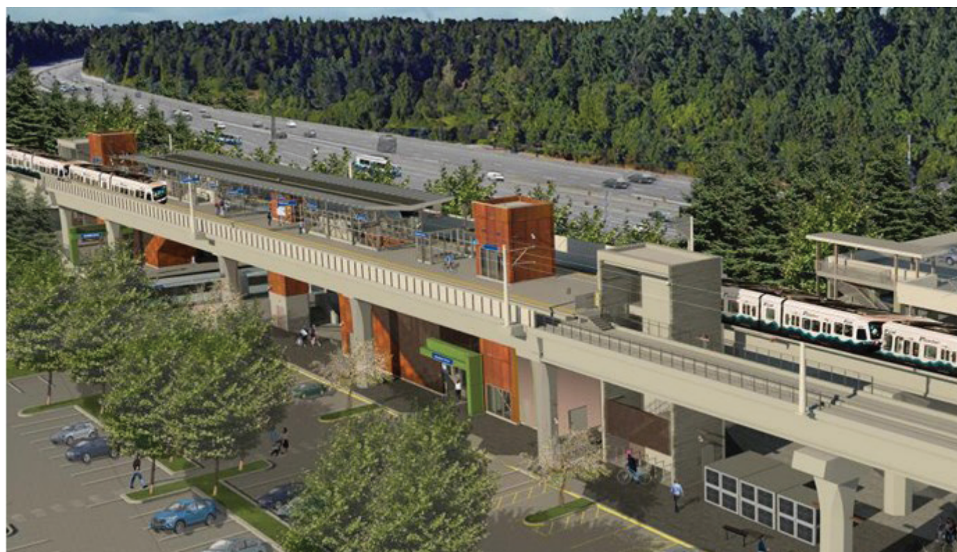
Light rail extension, Shoreline – Lynnwood, USA
