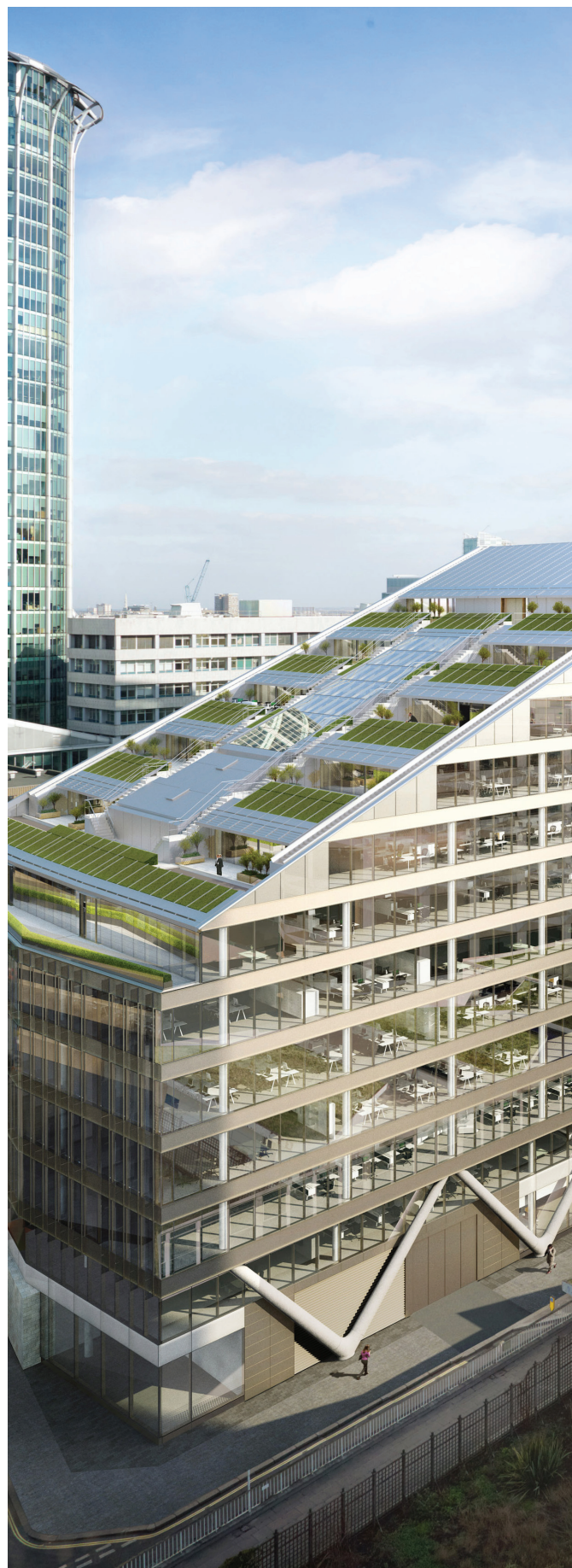
Moorgate Exchange project, London, U.K.
