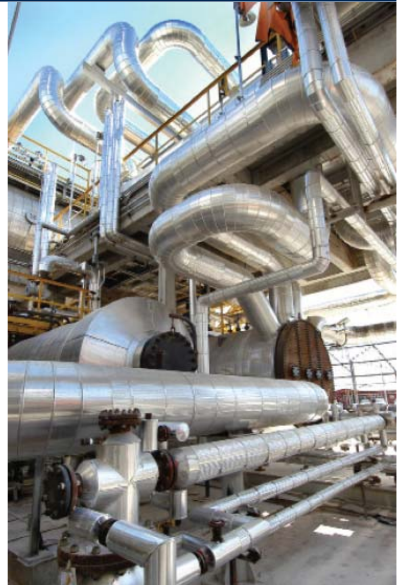
Petrobras, Brazil – Zero Accidents achieved
