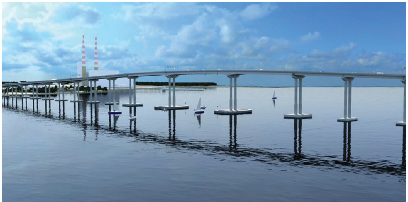
Bridge over the Potomac River, Virginia, USA
