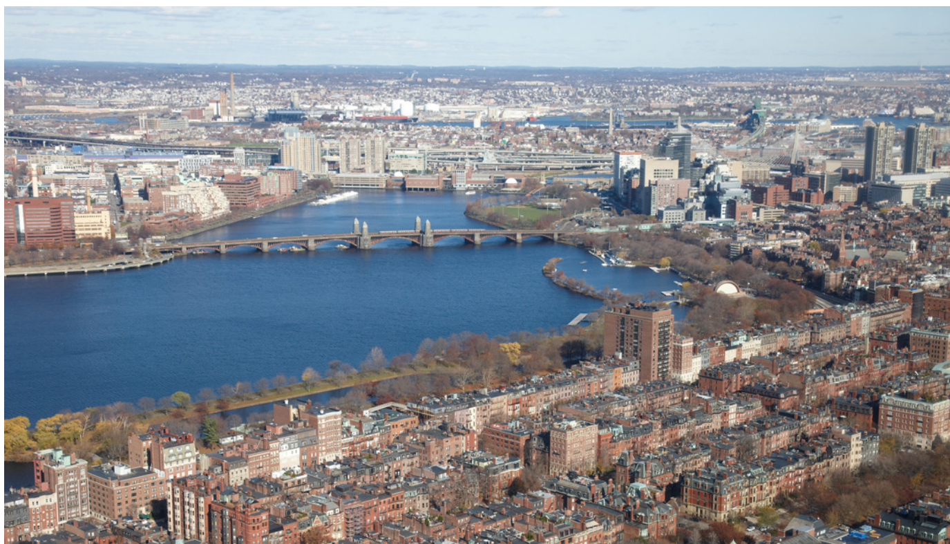
Longfellow Bridge, Boston, Massachusetts, USA.
