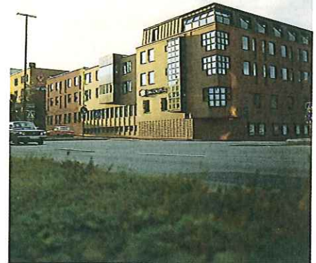
The Hotel Winn in Östersund, northern Sweden, was extended. The older portion is being renovated during 1987.
