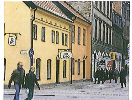
A historic house in Malmö, restored for Sulcus, a Skanska real estate company.
