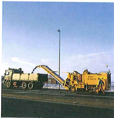
Asphalt paving with recycled roadway materials.
