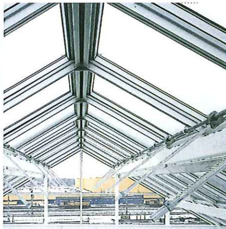
Glass superstructure at Skanska's office building in Älvsjö, near Stockholm.
