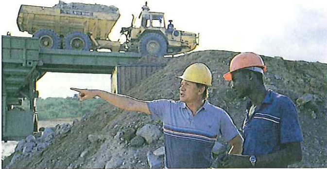
Access roads being built to the Kiambere power plant in Kenya.
