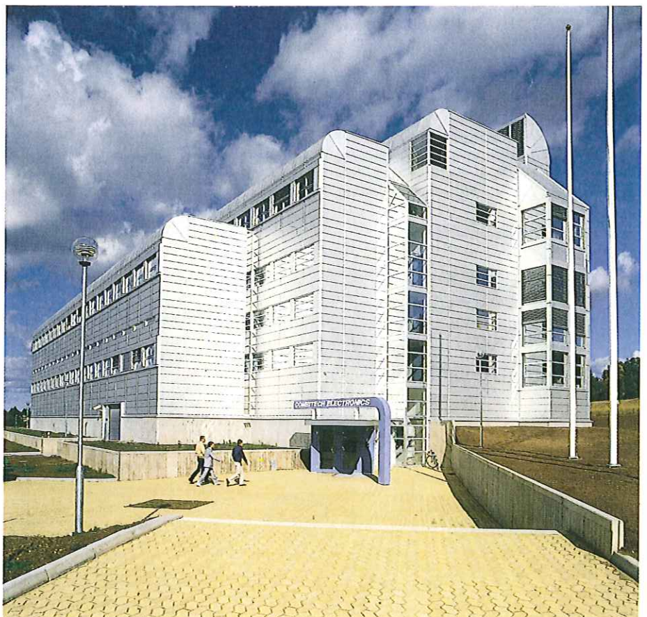
Saab-Scania Combitech's electronics factory and offices in Jönköping, completed in late 1986.
