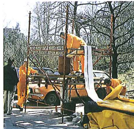
Restoration of old piping by the in-situ form method.
