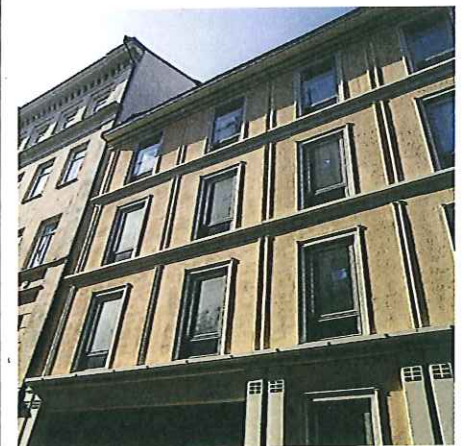
A new building in downtown Stockholm with a prefabricated façade blends into its surroundings.
