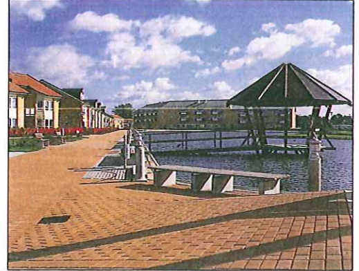
Paving stones at Lomma Centrum outside Malmö. Concrete paving stones in various designs and colors are one of Skanska Prefab's products.
