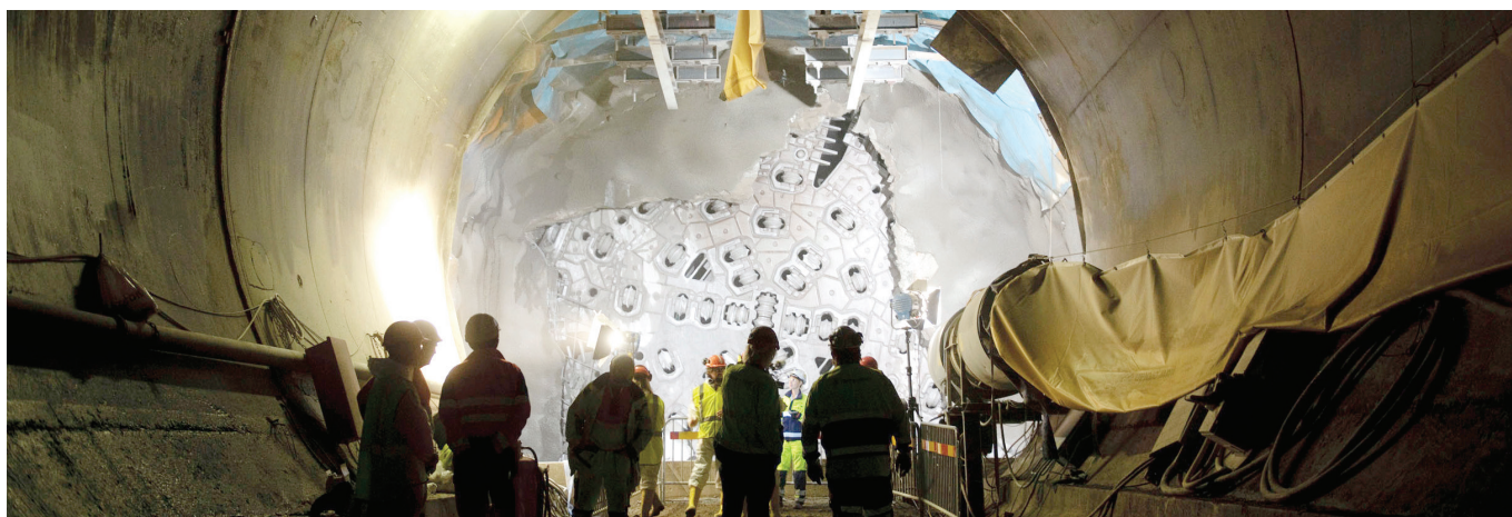
Breakthrough, Project Hallandsås, Sweden.
