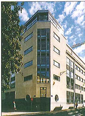
Gothenburg's new city court house was built by Skanska Väst for Skanska Fastigheter Väst, which owns the building.
