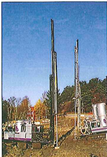
Stabilator has further refined its lime/cement column method for soil stabilization.
