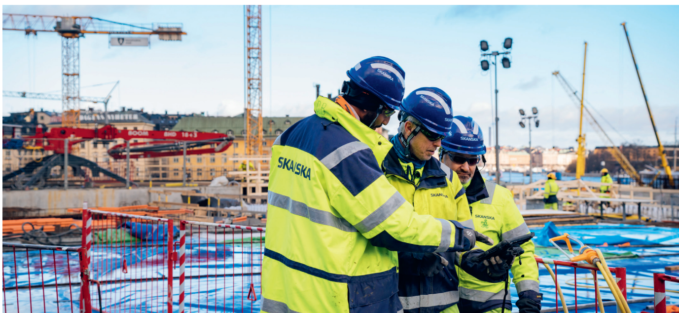
Digital tools on site, Slussen, Stockholm, Sweden
