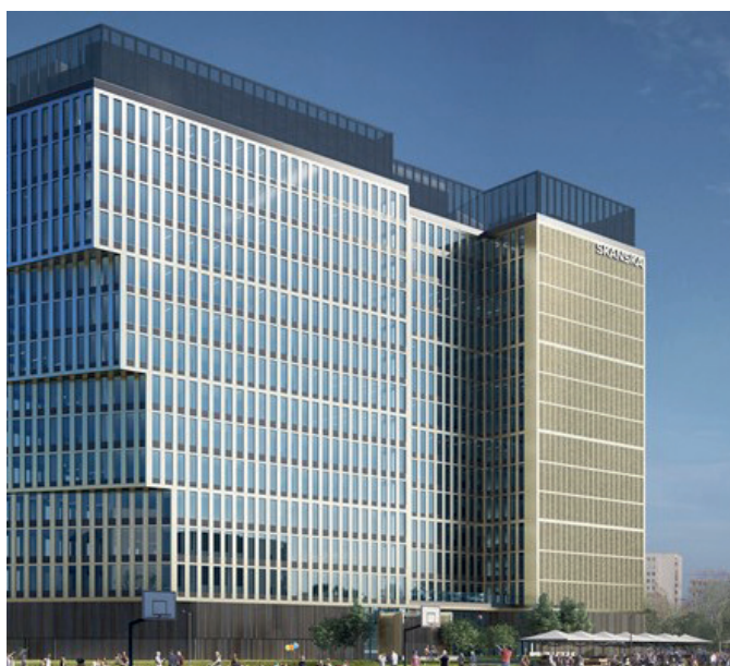
Investment, P180 office building, Warsaw, Poland
