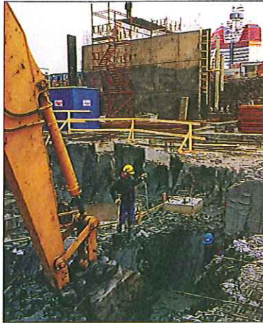
Several Skanska companies are involved in constructing the Gothenburg Opera in downtown Gothenburg.
