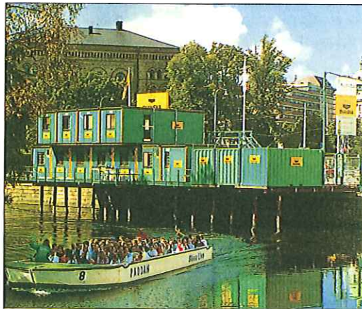
A creative work site configuration in central Gothenburg, where work sheds from Skanska Maskin were placed on pilings in the harbor channel.
