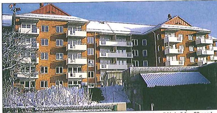
Near Jakobsbergs Centrum, a Stockholm suburban shopping center, JM is building 60 apartments for the Hästhoven cooperative housing association, intended for people aged 55 or over.
