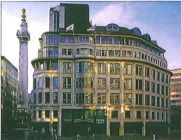
The 55 King William Street office property was designed to fit the architectural traditions of the City of London. Its copper roof and Portland stone façade also blend with the surroundings.
