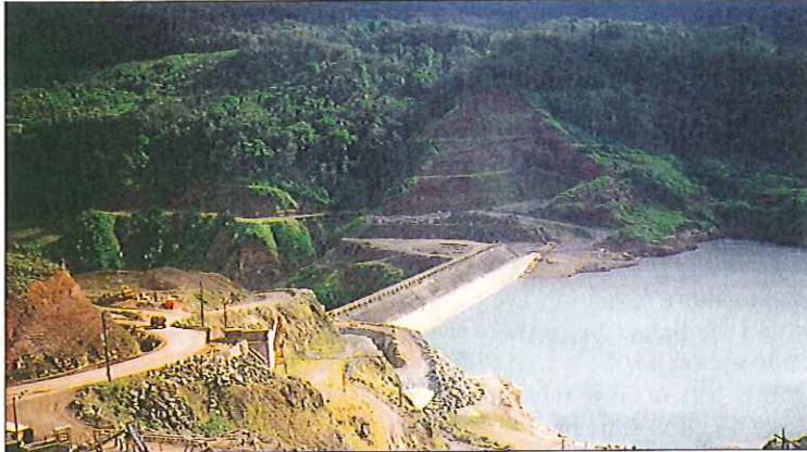
One of Civil Engineering's major projects is rebuilding the Fortuna hydroelectric power dam in Panama, increasing its height from 60 m to 100 m.
