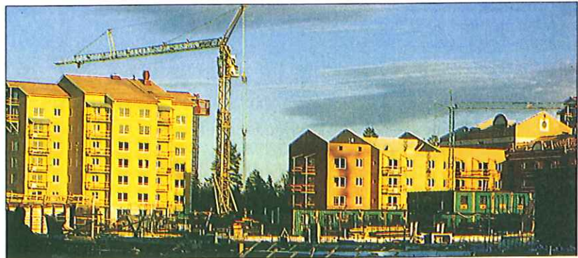
Skanska Prefab is supplying prefabricated building elements for 320 apartments in the Nydala Heights neighborhood of Umeå, which Skanska Norrland is producing on a design-construct basis.
