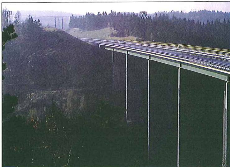
Skanska constructed two freeway stretches on the E6 European highway north of Gothenburg, including the 385 m (1,263 ft) long Ödsmål Bridge. Skanska Teknik was responsible for designing the bridge.
