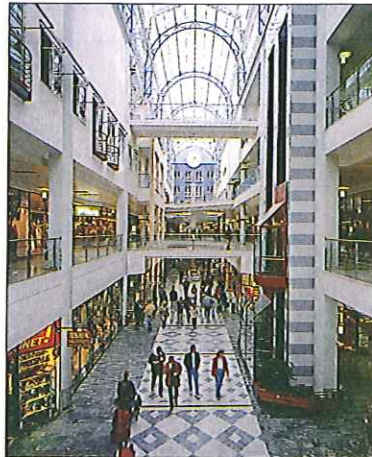
Under a contract with JM, Skanska Stålteknik manufactured and erected the frame for the new Täby Centrum north of Stockholm.
