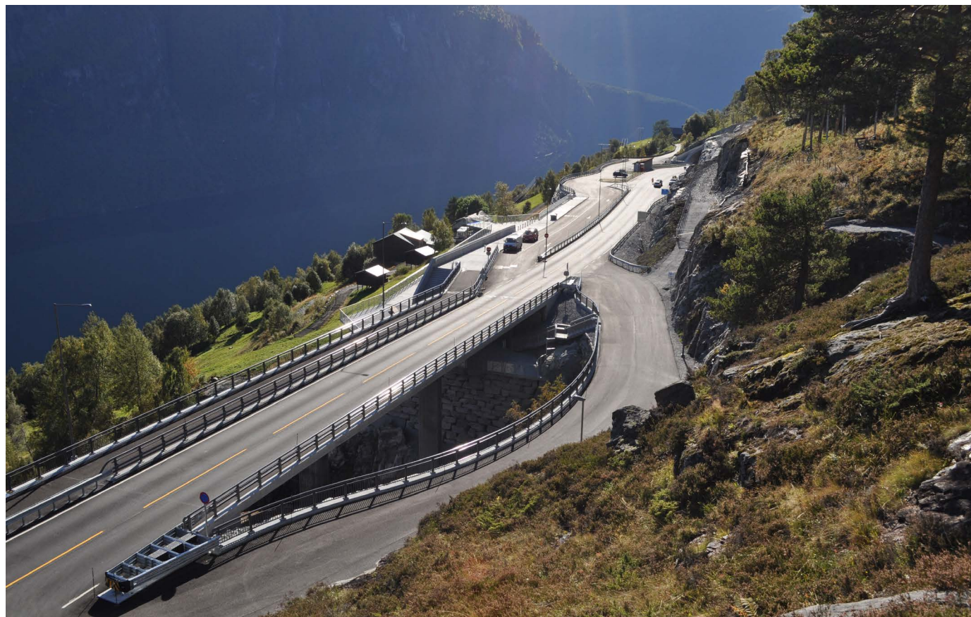
Streketunnelen, Stranda, Norway.
