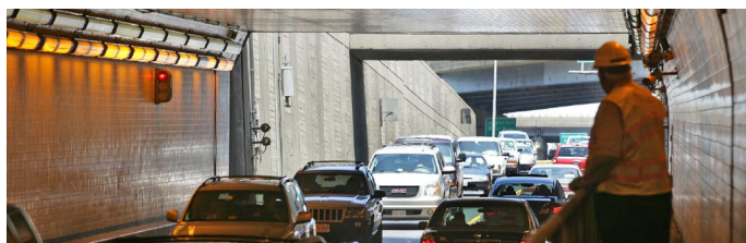
Elizabeth River Tunnels, Virginia, USA.
