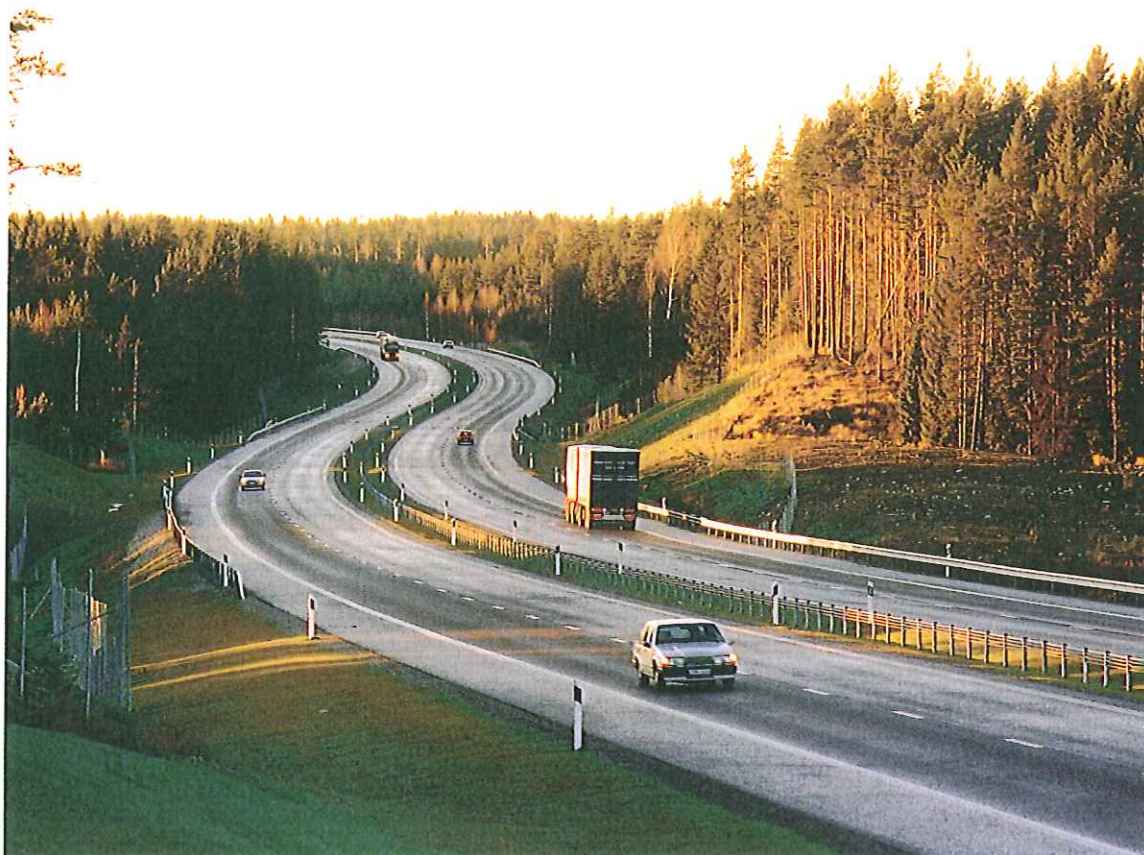
The new E4 free-way past Stavsjö, between Norrköping and Nyköping, was built to follow the contours of the landscape. Project time was shortened from three years to two.
