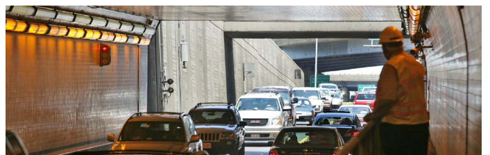
Elizabeth River Tunnels, Virginia, U.S.
