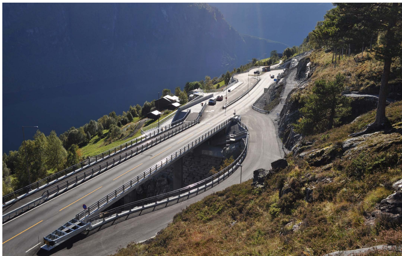
Streketunnelen, Stranda, Norway.
