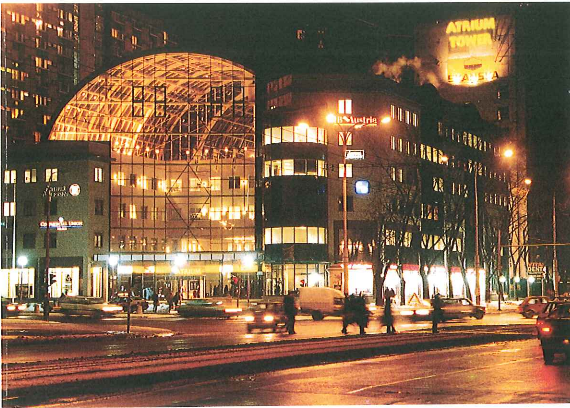
The second phase of the Atrium Business Centre in Warsaw, Poland is now under construction.
