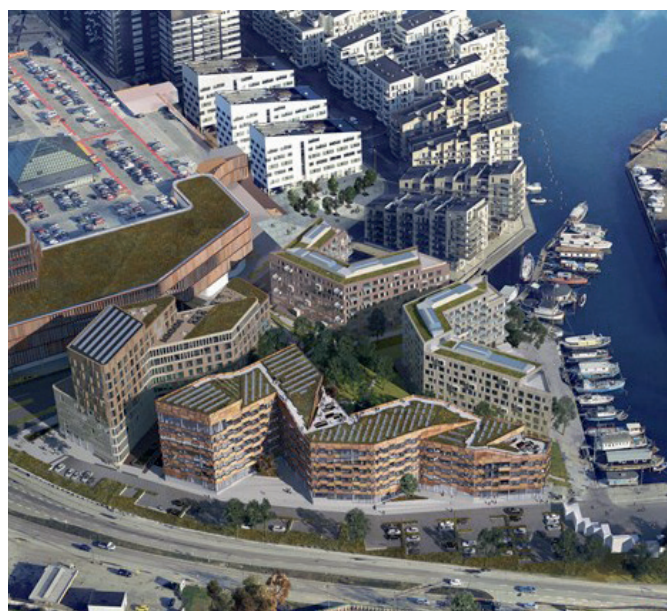
Divestment, CPH Highline, Copenhagen, Denmark
