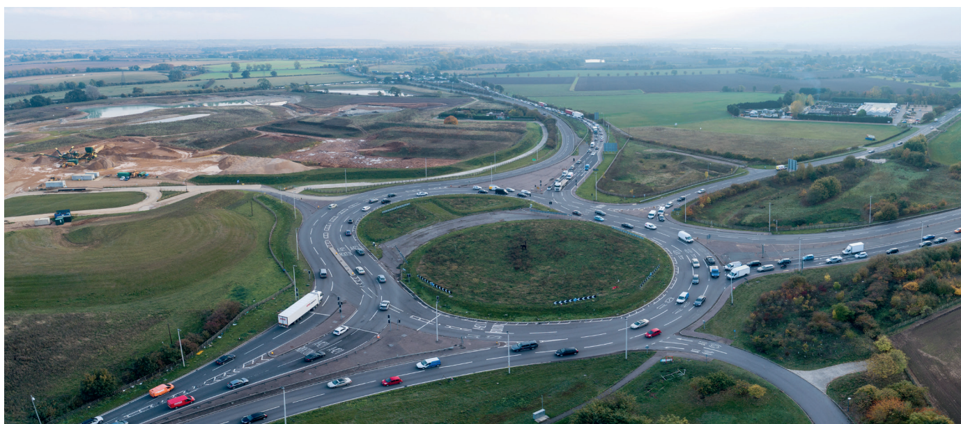
A428 road, East of England region, UK
