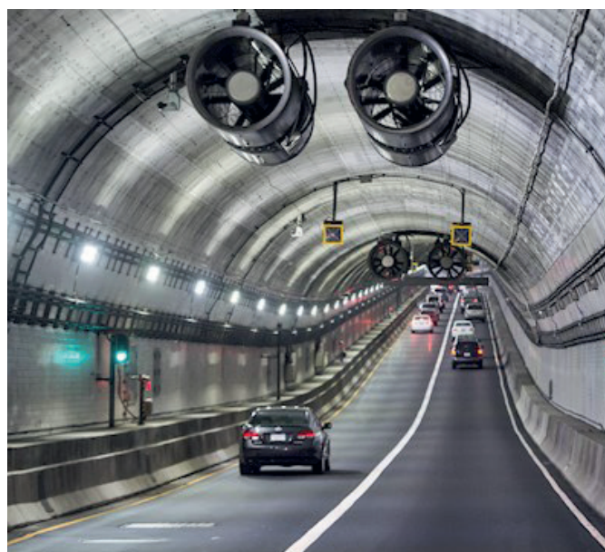
Divestment, Elizabeth River Crossings, Virginia, USA
