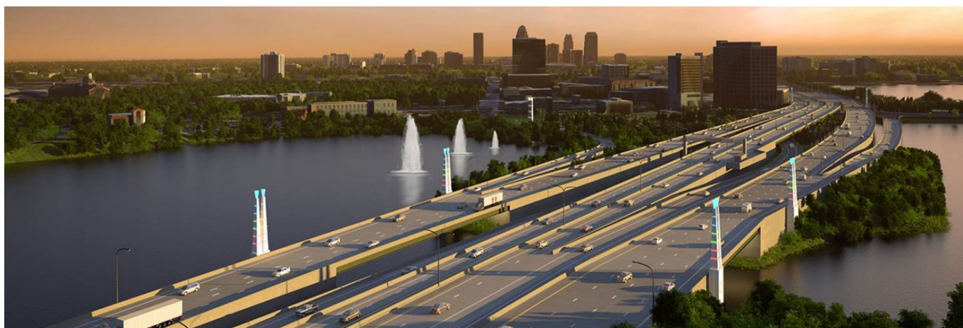
Interstate 4 Ultimate, Florida, U.S.
