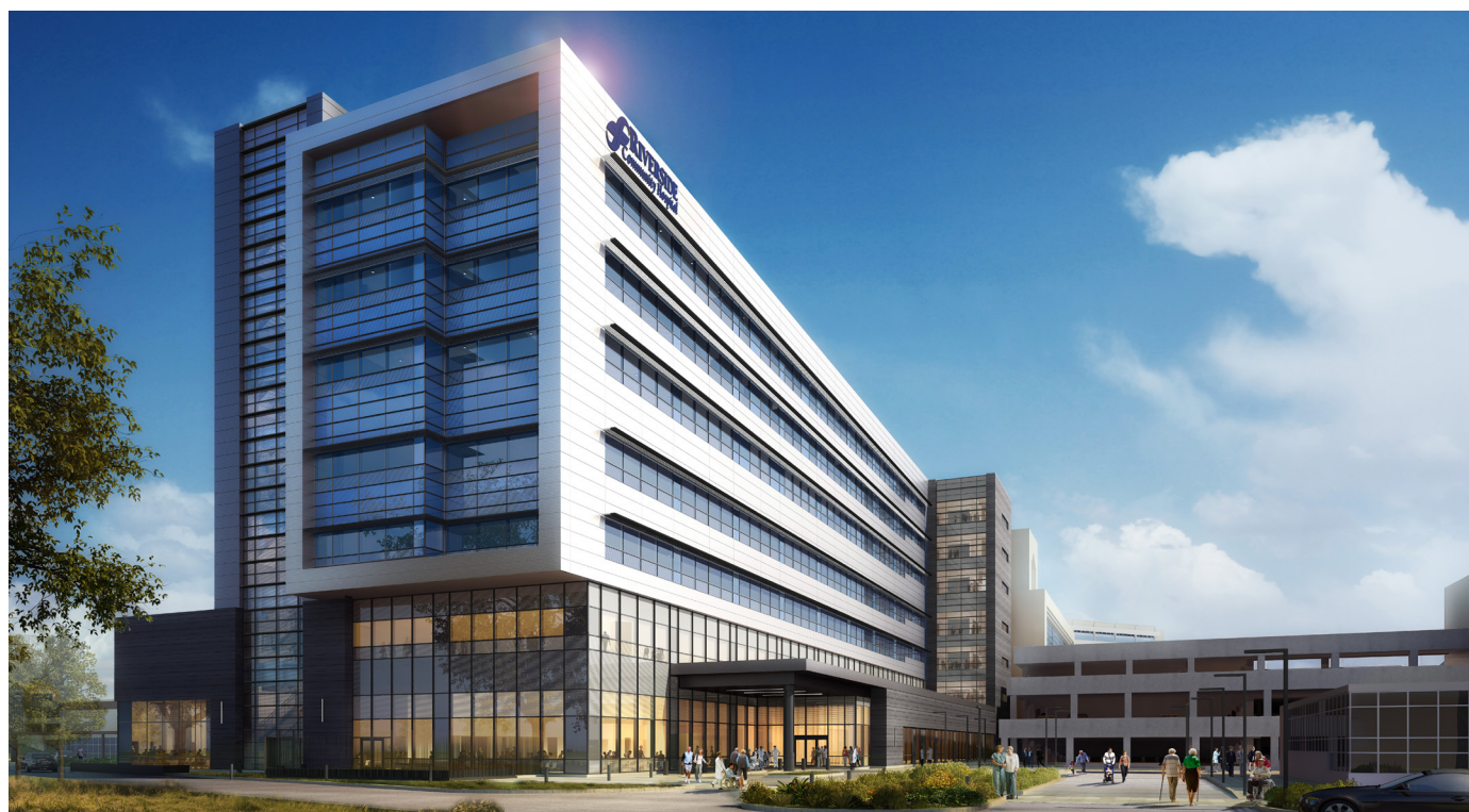
Riverside Community Hospital, Kalifornien, USA.
