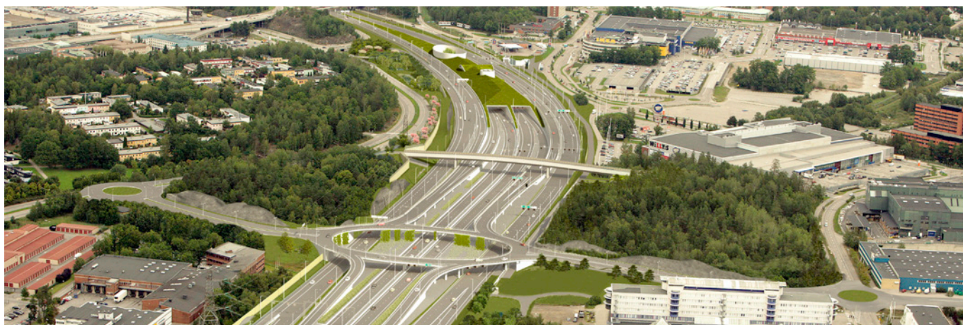
Stockholm Bypass Tunnel, Kungens Kurva, Sweden.
