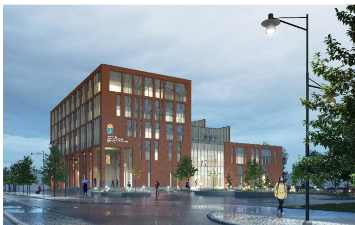
Investment and divestment, courthouse building, Växjö, Sweden
