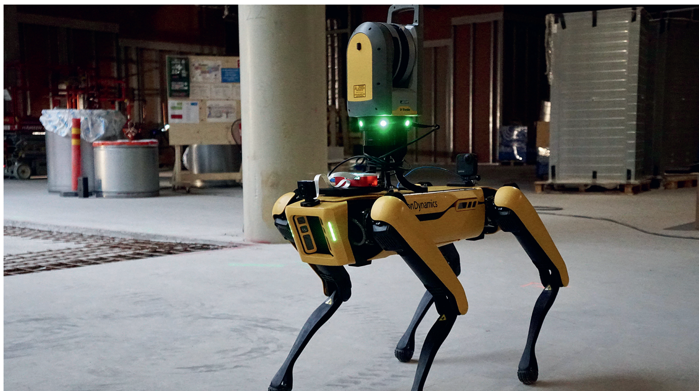
As part of Building 2030 consortium testing activities, Spot, the robot dog, visited Skanska's construction site, Lippulaiva Shopping Center, Espoo, Finland, to examine the feasibility of robotized reality capture for real-time construction management. Building 2030 consortium, including Skanska, develops a vision for the Finnish construction sector in the year 2030 to prepare for future changes in the field of construction to ensure a sustainable foundation for business in the sector going forward. Image: AE Partners.
