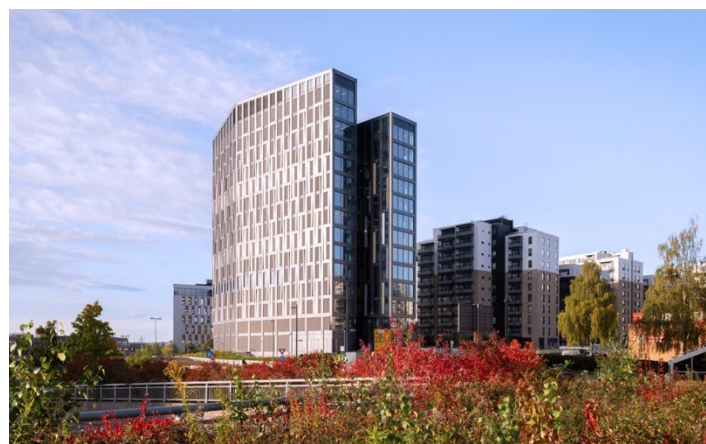
Divestment: Parallell, Oslo, Norway
