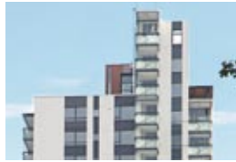
BIM used in planning work, Finland 31
