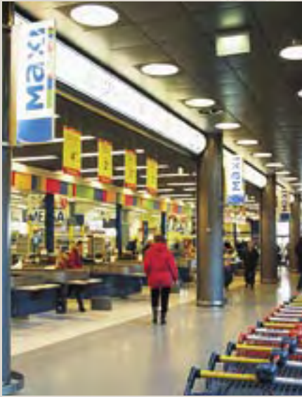
Currently under construction in suburban Helsinki is the second phase of the Sello shopping center in the Leppävaara district of Esbo. With some 170 stores and service premises due for completion late in 2005, Sello will be one of the largest retail centers in the Nordic countries. The first phase, including a department store, specialty stores, library and concert hall, was completed in 2003.
