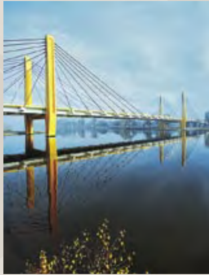
The Millennium Bridge across the Oder River is part of a new bypass highway around Wrocław, Poland. The bridge is 972 m (3,189 ft.) long in all, including a 290 m (951 ft.) central suspension span. The pylons are 50 m (164 ft.) high. The project was completed in less than three years.
