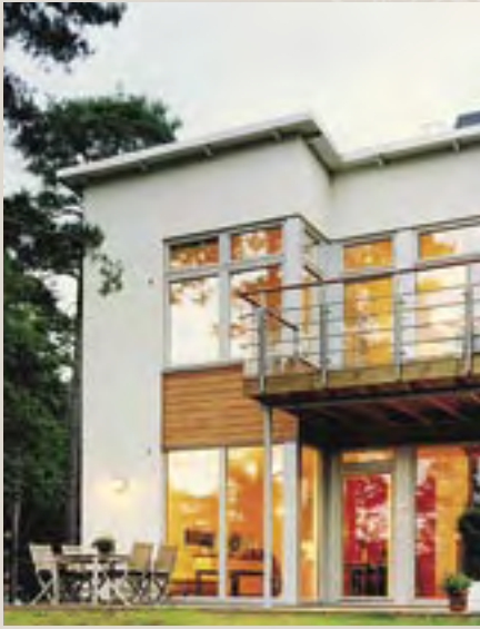
Trollåsen in Askim outside Gothenburg consists of 25 free-standing, individually owned single family homes that Skanska developed and built. Buyers appreciate both the design and location of the homes, most of them featuring wooded lots and sea views.
