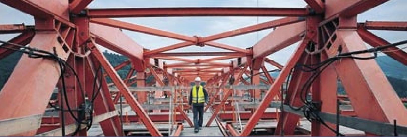
Poland has major infrastructure needs. The 600 m (1,968 ft.) long Milówka Bridge is part of an expressway in southern Poland. Skanska is the only construction company in Poland with access to the rolling scaffolding shown here, used in formwork of permanent bridge structures. Skanska is also responsible for building 90 km (56 mi.) of the A1 highway in northern Poland as part of a public-private partnership.
