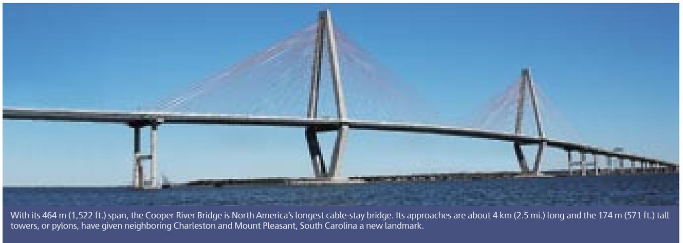
With its 464 m (1,522 ft.) span, the Cooper River Bridge is North America's longest cable-stay bridge. Its approaches are about 4 km (2.5 mi.) long and the 174 m (571 ft.) tall towers, or pylons, have given neighboring Charleston and Mount Pleasant, South Carolina a new landmark.
