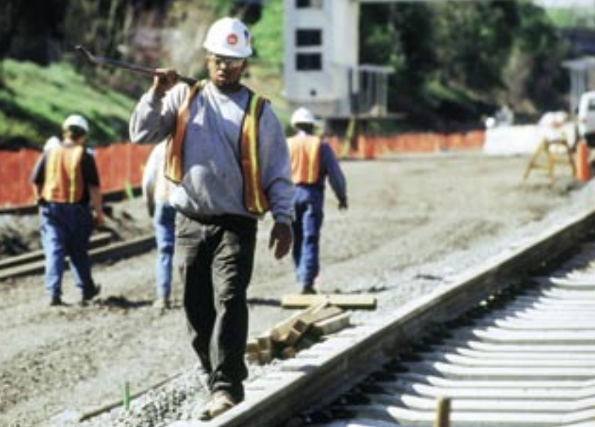
Highbridge Yard rail car service facility, New York City, U.S.A.
