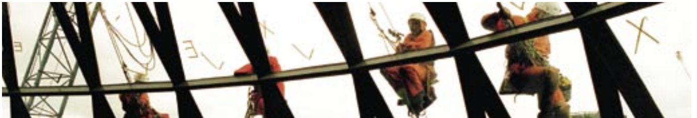
Swiss Re office building, London, United Kingdom
