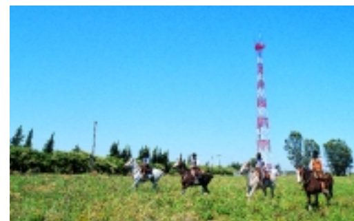
Expansion of infrastructure for mobile (cellular) telephone systems in Argentina.
