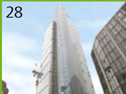
28 Heron Tower – tallest in the City of London
