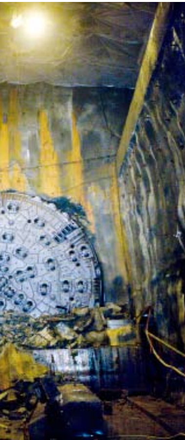
In August, a milestone breakthrough was achieved at the Hallandsås (Hallandsås Ridge) rail-tunneling project in southern Sweden. The tunnel-boring machine, named Åsa, completed the first of the two 5.5-kilometer pipes. The final breakthrough is planned for 2015.
