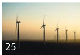
The Totoral Wind Farm generates green electricity in Chile
