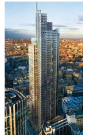
When completed in 2011, Heron Tower will rise to a height of 202 meters (663 ft.), making it one of the tallest office buildings in the City of London.
