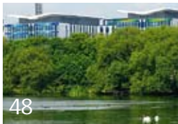
Europe's largest geothermal lake loop in Nottinghamshire, U.K.
