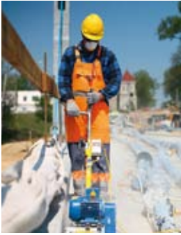
Building a bridge over the Pilica River, Poland.
