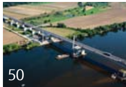
Phase II of the A1 expressway, Poland
